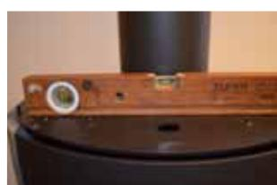
**9:** Check that the steel platform is screwed down as far as possible and that it is level.
