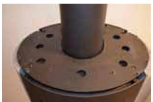
**8:** Place the steel platform on the 4 or 5 special nuts on the top of the stove.
