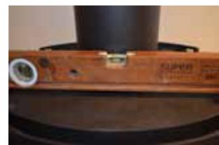
**7:** Check that the wood-burning stove is level. If necessary, mount/adjust the 4 adjustable feet under the stove itself so that it stands stable and safely on the base. **NOTE! There must be a minimum of 8 mm air under the wood-burning stove if you would like to mount a Termatech form cut glass plate.**
