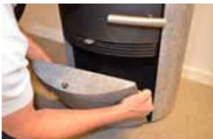
**24:** Carefully mount the stone with the gasket side downward in the combustion compartment and press the peg on the top down, so that it can fasten in the hole on the ribs, set it carefully in place.
