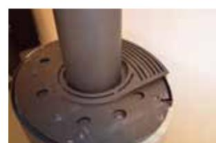
**11:** Now mount the rear soapstone (Note that the front and rear stones are identical, so if you think that one of the stones is "nicer looking" than the other, then mount the "nice looking" stone in the front and the other to the rear) In the under bottom edge of the stone there are 4 holes that must fit down in the 4 corresponding guide pins on the steel platform.
